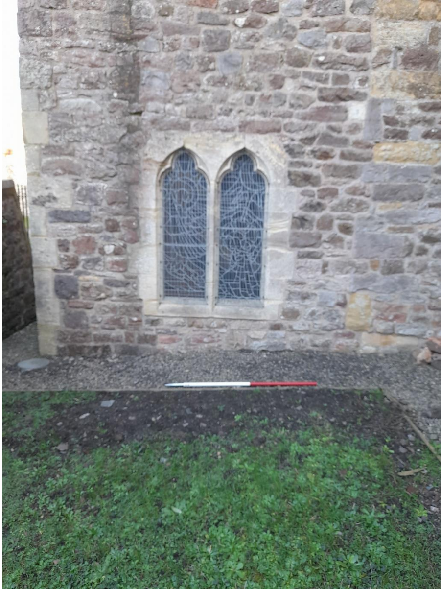
Figure 3. The backfilled lightning conductor trench looking eastwards towards the west wall of the north aisle. The connecting wire trench may be seen extending from the south end of the trench to the west (bottom-right in this photograph). The connecting wire trench was excavated to a depth of c. 200mm, within the dark/brown-black, humic, topsoil (001). The ground surface slopes gently downwards from south to north, from 12.48m OD to 12.35m OD (as surveyed by dumpy level from the Benchmark located on the western face of the church tower, recorded on the OS sheets as at 41.69 feet ODN or 12.71m ODN).
